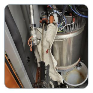
2 You can hang a small bucket on the inlet of the heat exchanger to catch any scale that may come out of the heat exchanger coil.
