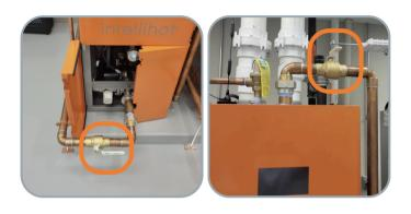
2 Using the T&P Relief valve, release any excess pressure inside the unit.
