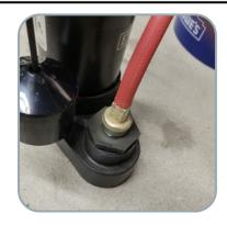
2 Thread a 3/4" MH x 3/4" FIP Adapter on the inlet and the outlet elbows.
