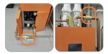
Once the pump is bled, turn on the unit at the rocker switch and check the flow rates on each heat exchanger. You should be seeing about 4 or 5 gpm on each hex.
