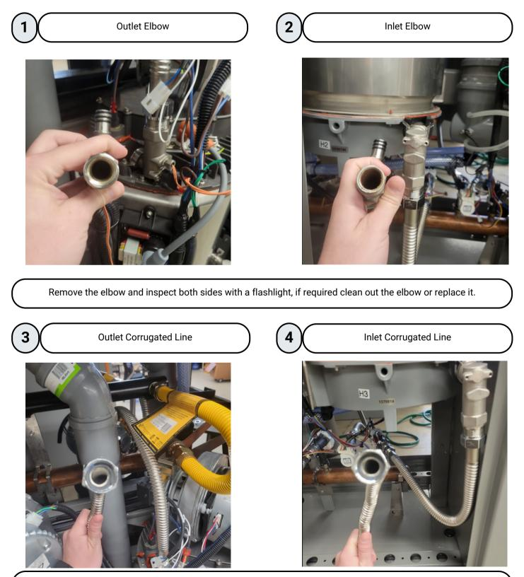
Remove the corrugated line and inspect for any blockage or buildup, and clean out if required.
