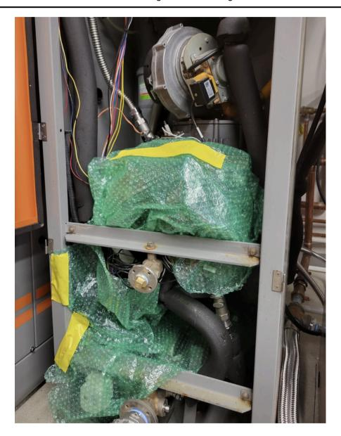
Begin the descaling process with the bottom heat exchanger, when moving to the top heat exchanger leave the bottom heat exchanger covered. As well ensure that the bottom blower is covered when descaling the top heat exchanger.
