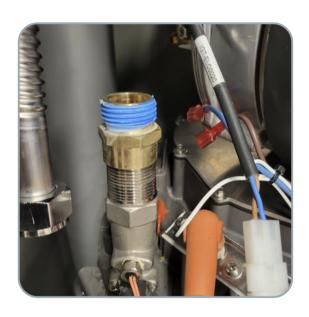
Connect one of the hoses to the outlet of the sump pump and then to the inlet elbow of the heat exchanger.
