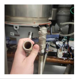
Remove the elbow and inspect both sides with a flashlight, if required clean out the elbow or replace it.
