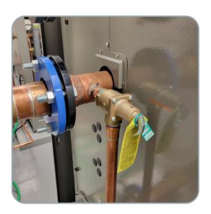
Using channel locks unscrew the 3/4" cap on the inlet side of the unit, and attach the garden hose to the open port, and let the water drain out.
