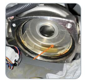
**2** Screw in the 4 bolts that hold the pump cartridge on the silver volute. Ensure that the connection for the electrical box is facing up.
