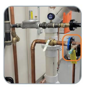
Isolate the unit by closing off the inlet and outlet isolation valves.
