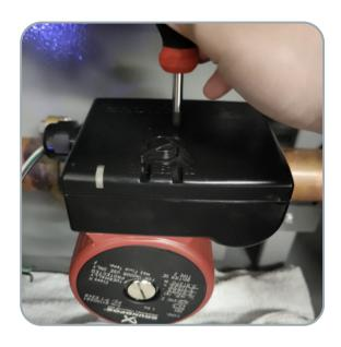
Using a stubby flat head screwdriver loosen the bleed screw on the pump about 3 turns, and let any air bleed out of the pump. Be prepared with some rags as water may drip out.
