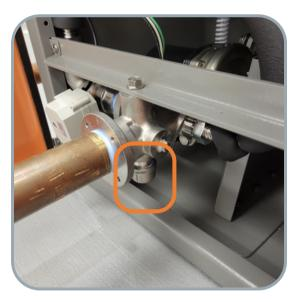
Slowly open up the outlet isolation valve then slowly open up the inlet isolation valve
