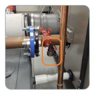
Using a flat head screwdriver loosen the bleed screw on both pumps about 3 turns, and let any air bleed out of the pump. Be prepared with some rags as water may drip out.
