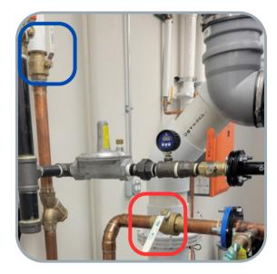
3 Using the T&P Relief valve, release any excess pressure inside the unit.
