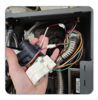
Install the water valve onto the inlet strainer and install the clip to hold them together.
