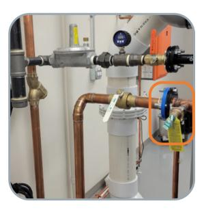
**2** Isolate the unit by closing off the inlet and outlet isolation valves.
