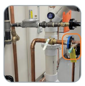
2 Isolate the unit by closing off the inlet and outlet isolation valves.
