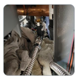
4 To ensure that the clips are connected correctly try to spin the clip around and it should spin 360 degrees
