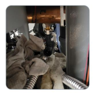
Insert the inlet corrugated line into the short end of the water valve and install the silver clip to hold them together
