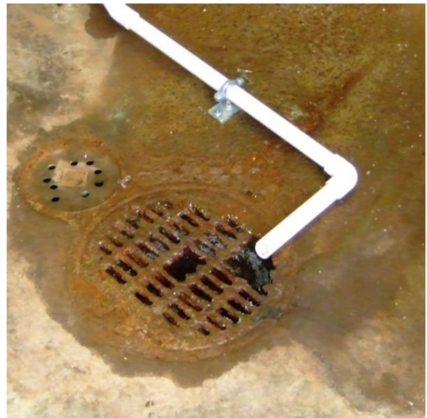
Figure 3 - Drain corroded by acidic condensate.
